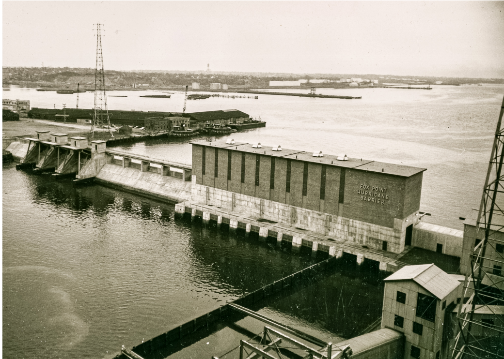
Figure 5.1: The Fox Point Hurricane Barrier following completion in March 1966 (Providence, Rhode Island). Photo taken by the New England Division of the U.S. Army Corps of Engineers (Waltham, Massachusetts).
