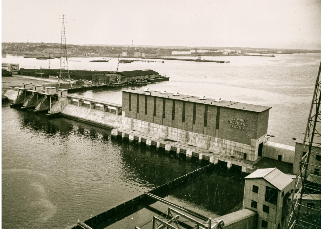
Figure 6.2: The Fox Point Hurricane Barrier following completion in March 1966 (Providence, Rhode Island). Photo taken by the New England Division of the U.S. Army Corps of Engineers (Waltham, Massachusetts).
